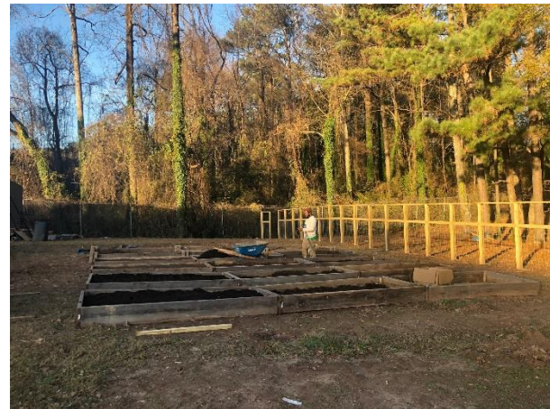
Getting fencing ready for livestock
