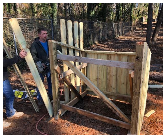
Constructing our Goat House
